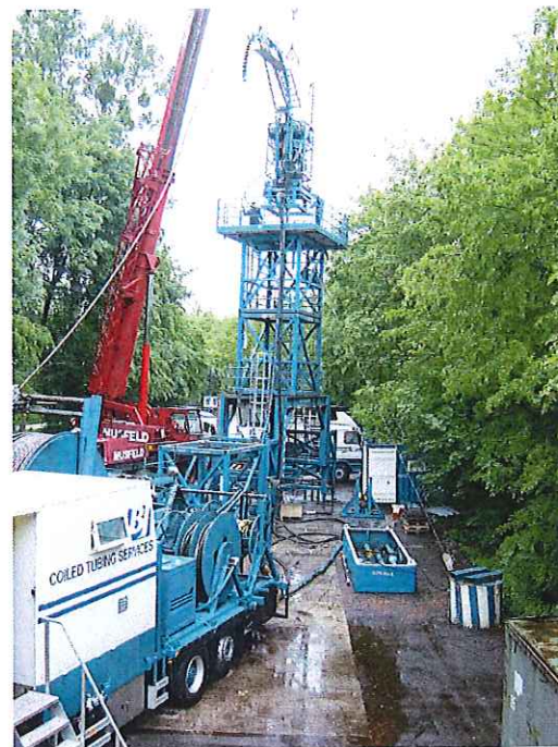
Figure 6. Coiled tubing unit
