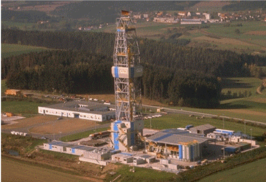
Figure 2-2. Deep drilling rig UTB-1 GH 300 EG.
