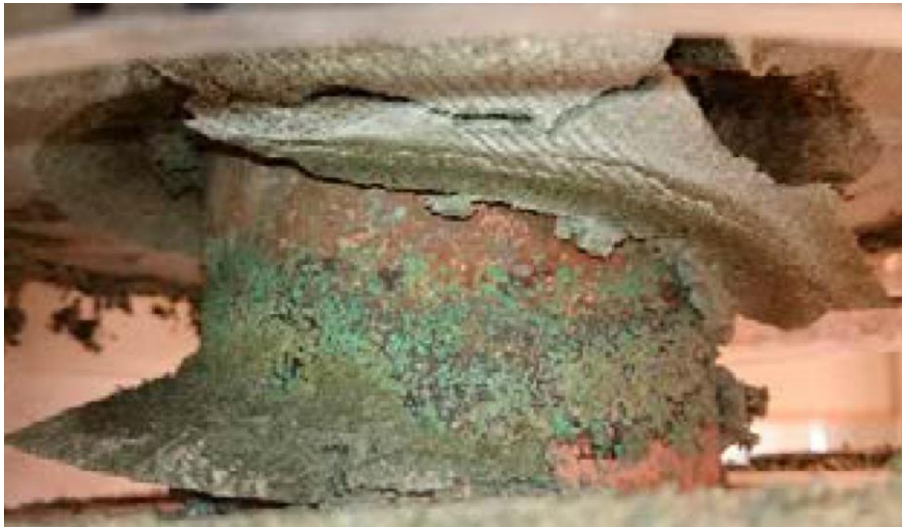
Figure 2.8. Detail from Figure 2-27 in TR 15-09. Severe corrosion of the copper heating tube after only seven days of laboratory exposure that at least reminds of the true Sauna effect, i.e. with only indirect contact with 0.6M chloride solution.
