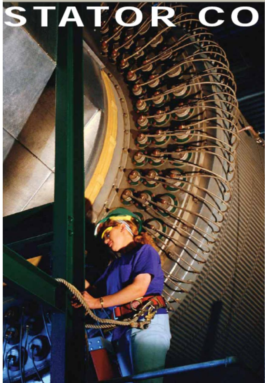
Corrosion in the stator cooling system of power generators is a primary source of maintenance costs and plant downtime.
